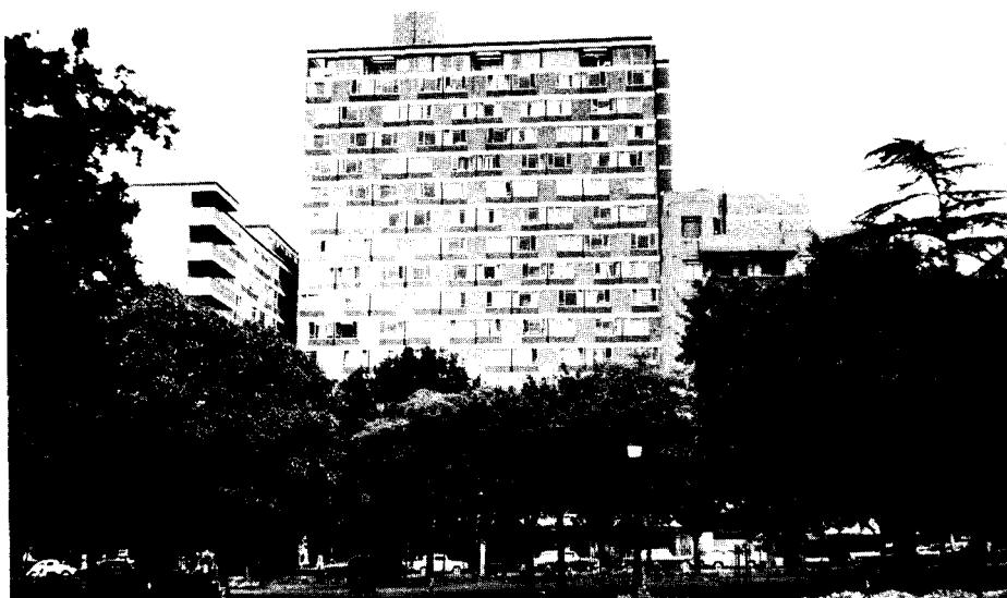
Windsor Gardens, Johannesburg, South Africa. In these 17th-floor penthouse offices, the Work of God in South Africa is carried on.
